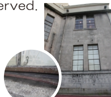
Window frames bent by the blast
